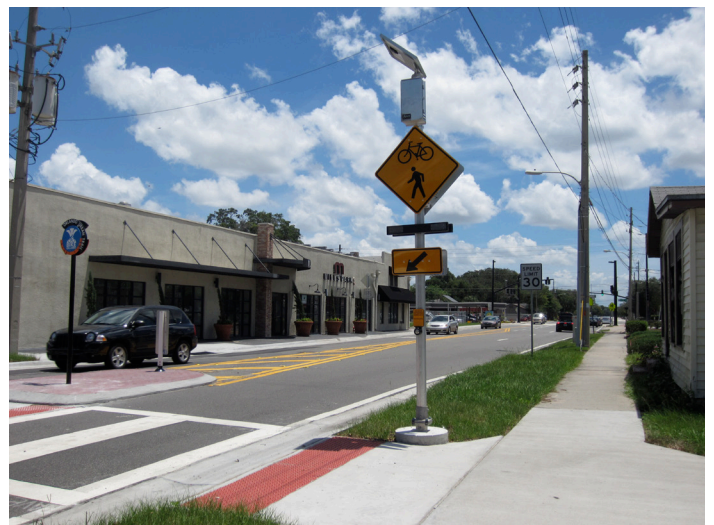
RRFB signal at ped crossing
