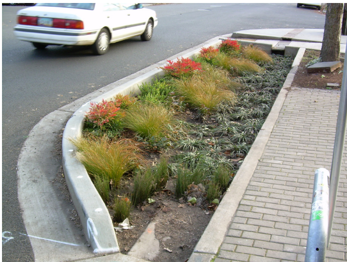
LID bulbout stormwater planter
