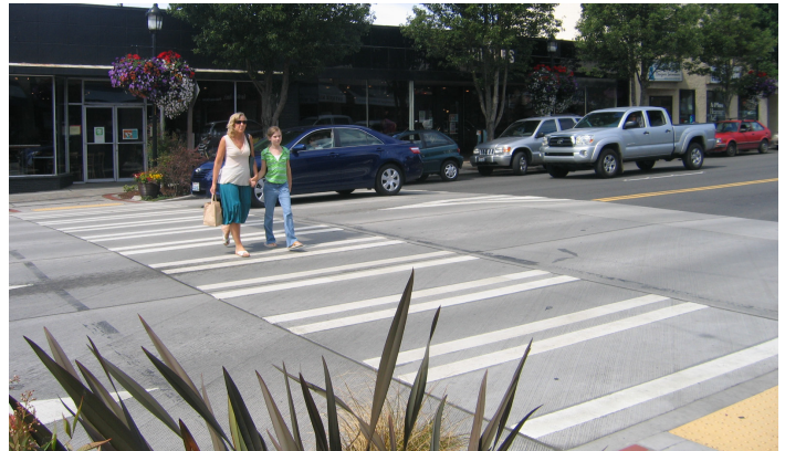
Raised mid-block crossing
