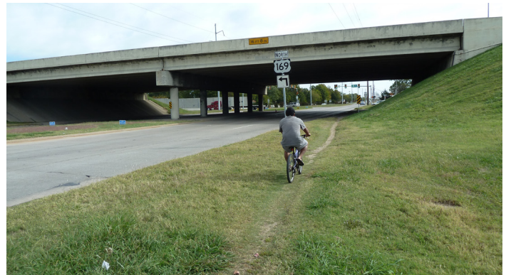
No sidewalks along E 21st Street under Hwy 169
