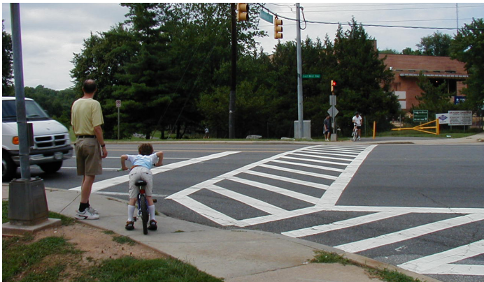
High visibility crosswalk at intersection
