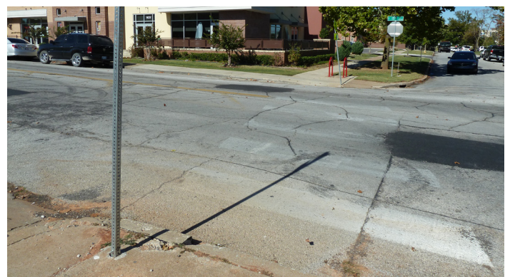
Lack of quality crosswalks along 15th Street
